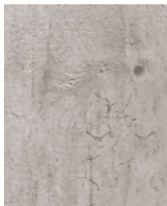
MW22 - Coarse Concrete F163 FS
